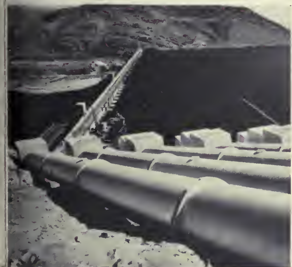
OVER THE HILL —Columbia River water will climb through the huge pipes shown immediately above. The air photo shows what will happen when the first pump starts at Grand Coulee Dam. The first pump unit, located deep inside the pumping plant (drawn in foreground) will start turning as power feeds from the L-1 generator in the left powerhouse. Water will surge up the discharge pipe, for right on the hill, into the winding Feeder Canal (center of photo). The Columbia River ultimately will fill the Grand
